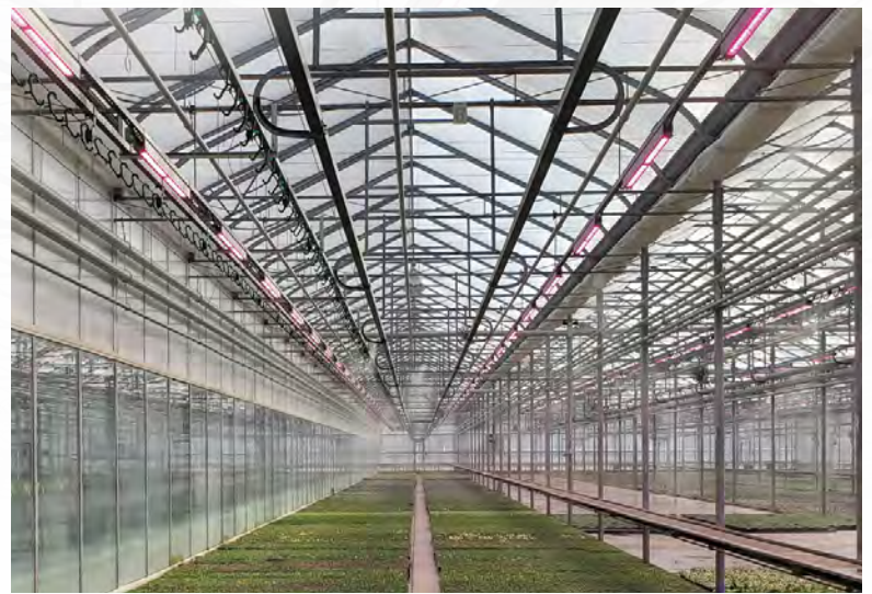
Most high-intensity light-emitting diodes (LEDs) emit very little far-red light, but there can be compelling reasons to include far-red in a light spectrum.
